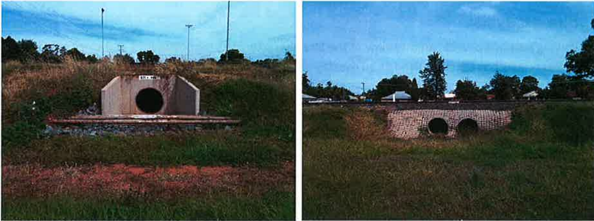
PHOTOS OF CULVERTS UNDER THE RAILWAY LINE ADJACENT TO THE SITE (LEFT: NORTH-WEST CULVERT; RIGHT: SOUTH-EAST CULVERT).
