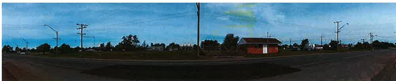
PHOTO (PANORAMIC) LOOKING SOUTH-WEST ACROSS THE HIGHWAY TOWARDS THE SITE.
