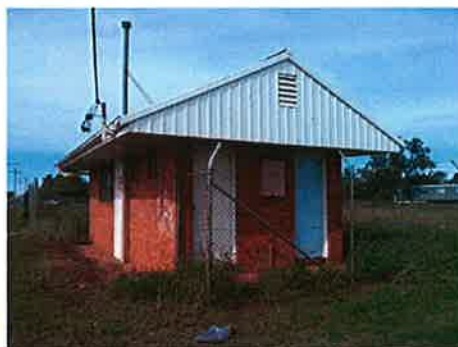
PHOTO OF OLD FUEL DEPOT BUILDING
